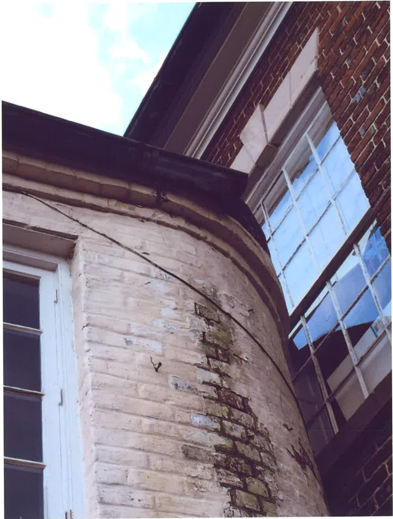
Photo 4 Current detail of exterior wall of curve and intersection with original rear wall of dwelling
