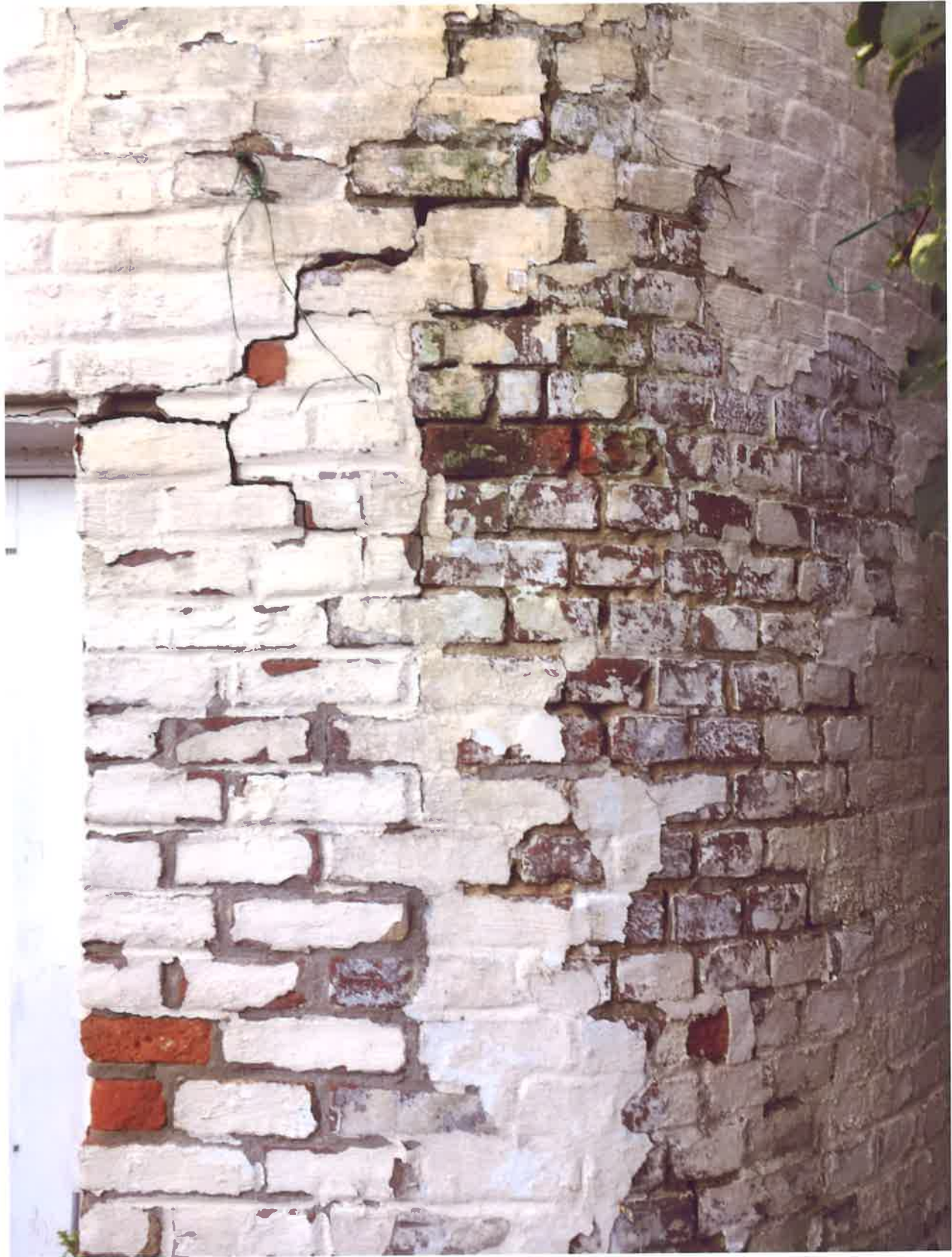
Photo 5 Current detail of exterior wall of curve
