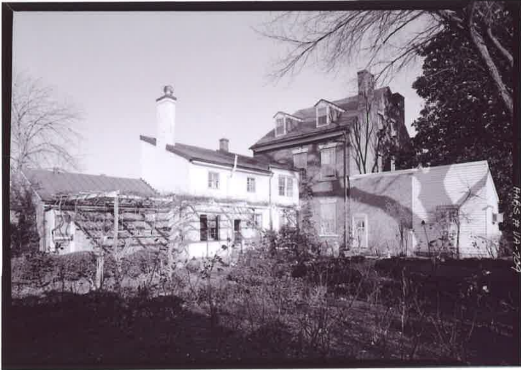
Photo 1 Overall of rear of house from HABS Records
