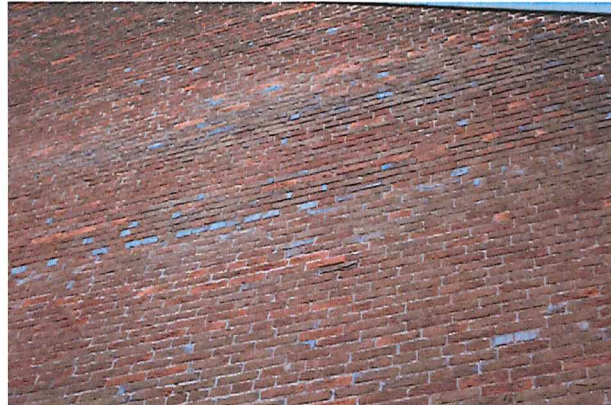
4 NORTH ELEVATION - REPOINT JOINTS NOT TO SCALE
