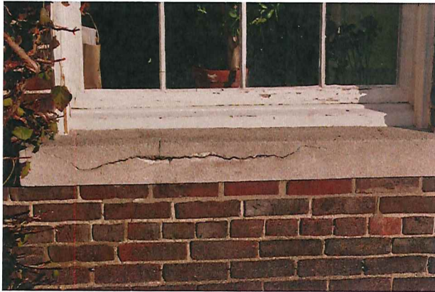
1 CONCRETE SILL - REPLACE NOT TO SCALE
